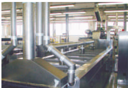
Industrial vessels and storage tanks
